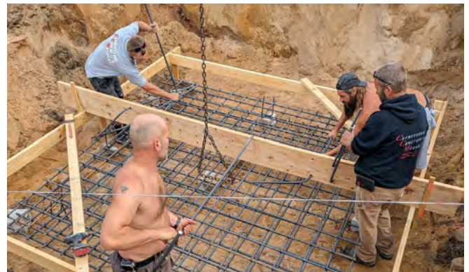
Cornerstone crew ties steel for the foundation of the Ivy Walls
