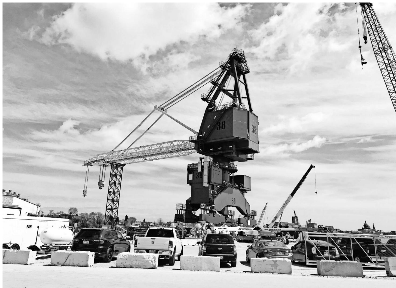
A giant crane that will lift 140-ton loads for the U.S. Navy was built by Konecranes and Broadwind Heavy Fabrications in Manitowoc. PATTI ZARLING/USA TODAY NETWORK-WISCONSIN
