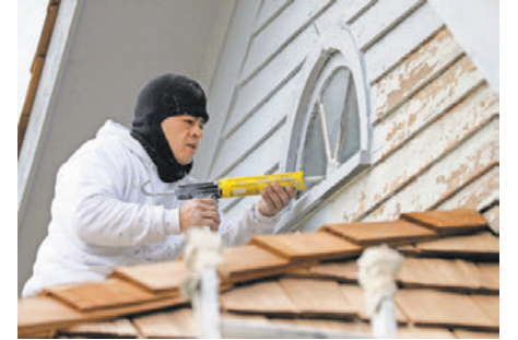
Investing in weather stripping or caulking can seal air leaks that may be releasing heat from your home. MIKE DE SISTI / MILWAUKEE JOURNAL SENTINEL
