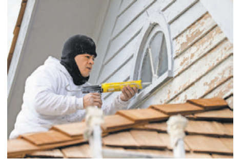
Investing in weather stripping or caulking can seal air leaks that may be releasing heat from your home. MIKE DE SISTI / MILWAUKEE JOURNAL SENTINEL
